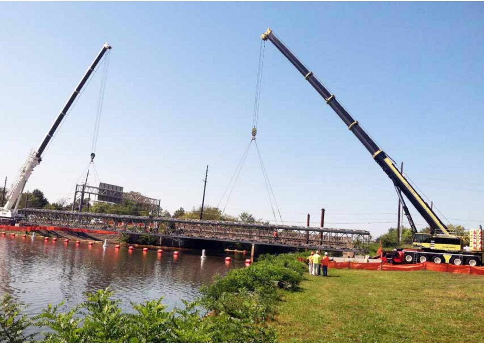
A 221 foot long pedestrian bridge in New Jersey being lifted into place using two cranes.
