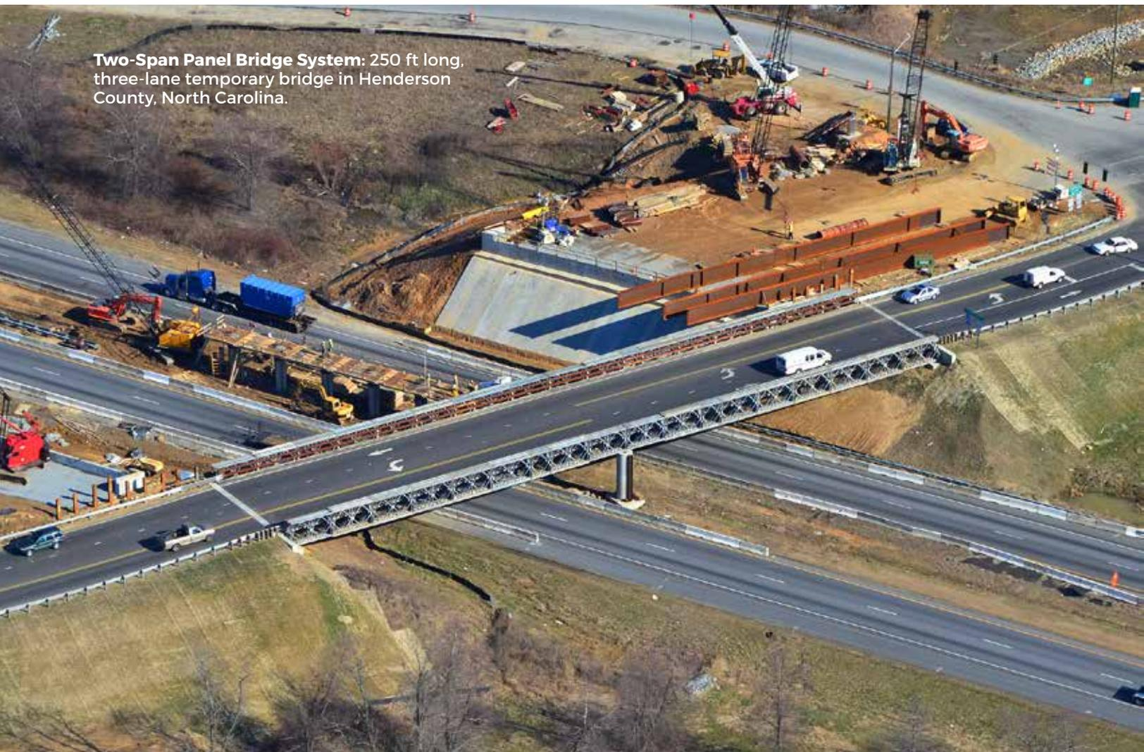
**Two-Span Panel Bridge System:** 250 ft long, three-lane temporary bridge in Henderson County, North Carolina.
